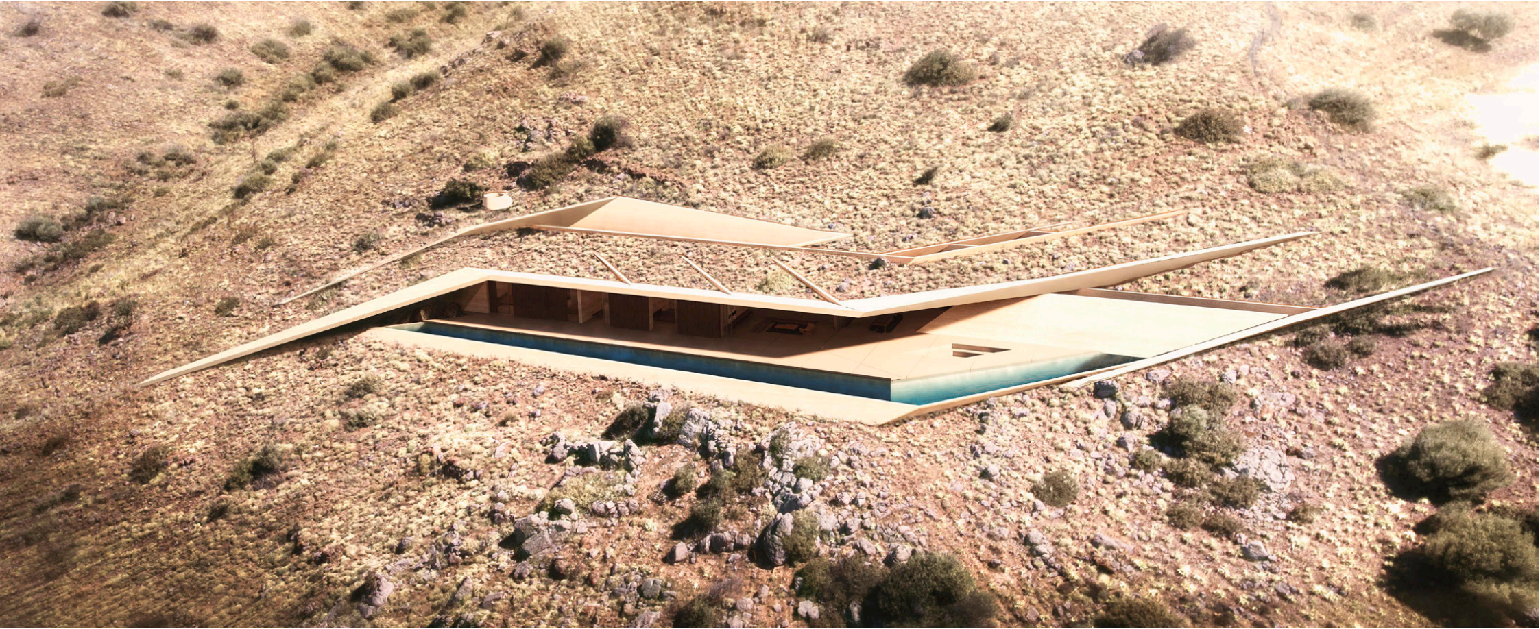
View from the South
